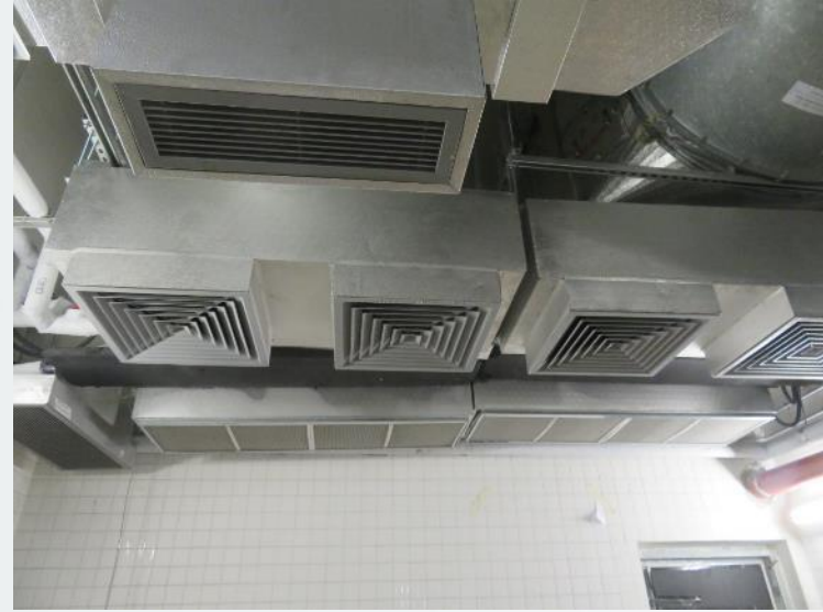
Sprinkler heads were obstructed by ductworks
