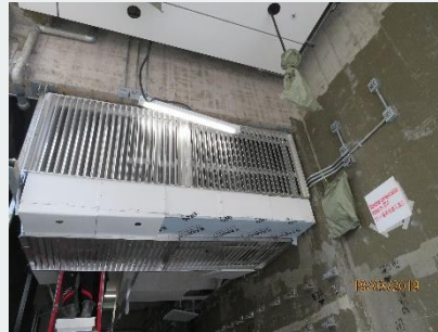
Pressurization of Staircase
