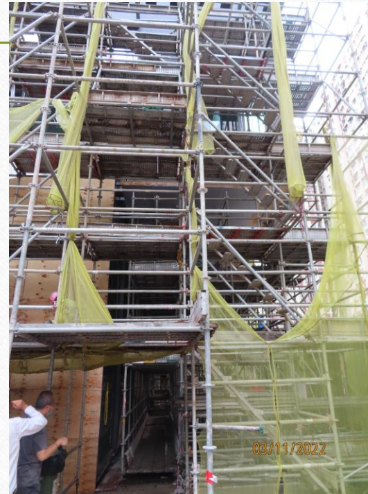
Extensive Scaffolding within inspection area
