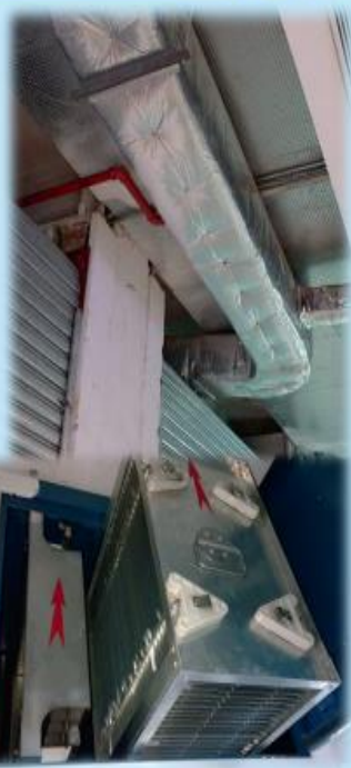
防火漆 / 溶液處理 Fire Retardant Paint / Solution Treatment
