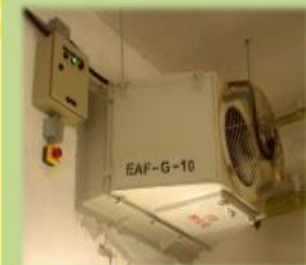
排煙系統 Smoke Extraction System
