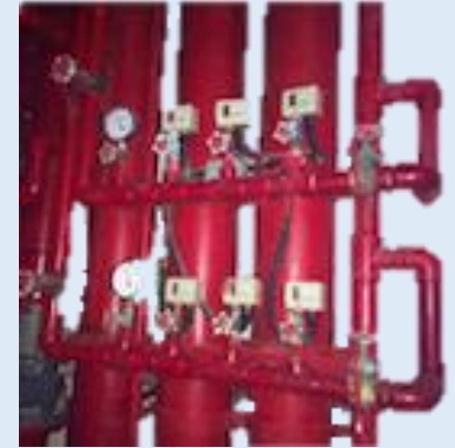
Water Columning Prevention Device(s)
