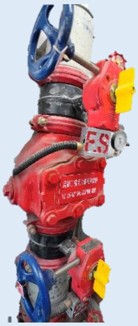
Sprinkler Control Valve
