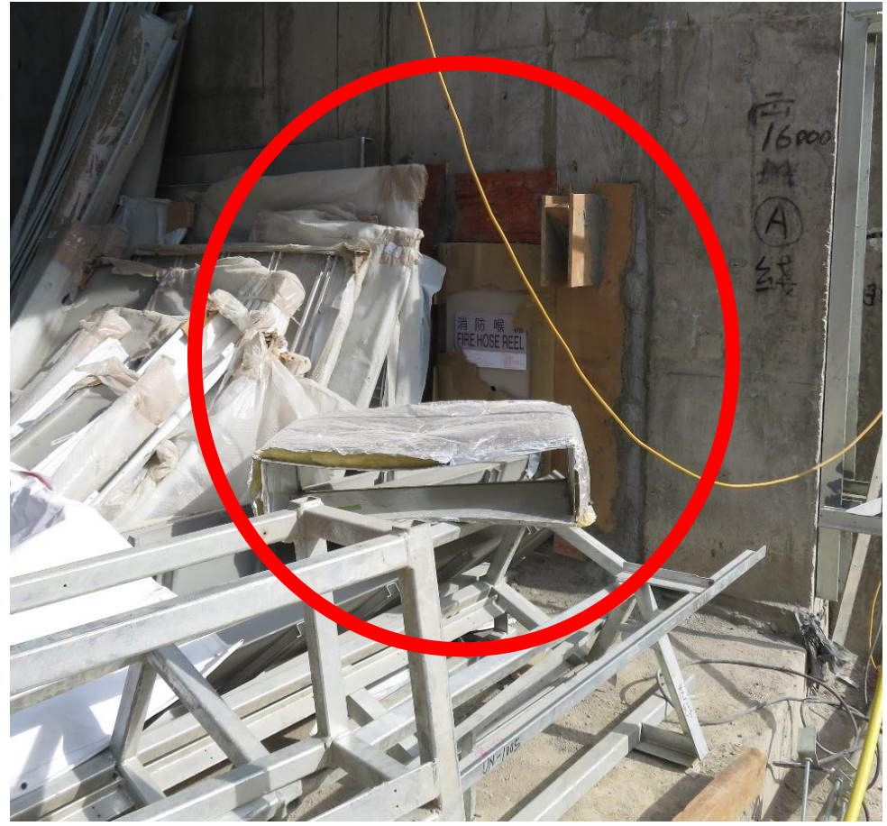
FS inlet & Hose reel were blocked
