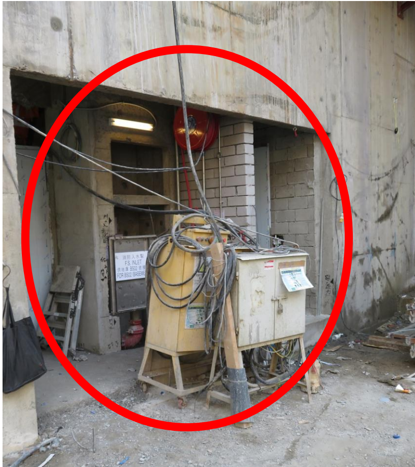
FS inlet & Hose reel were blocked
