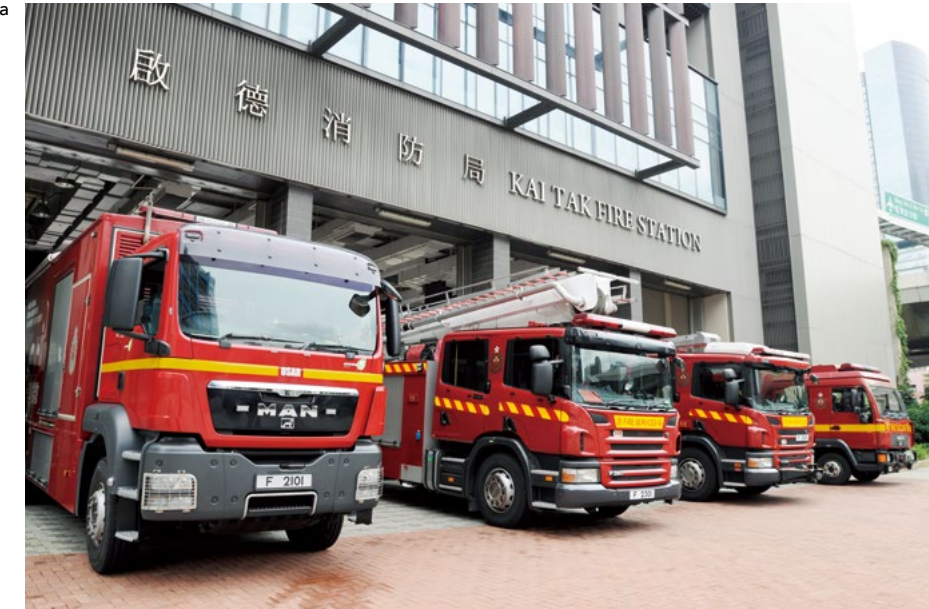
a 消防局及救护站分布于全港各区的策略位置，务求在不同地区发生紧急事故时，都能在相应的规定／目标召达时间内派员到达现场处理。 Fire stations and ambulance depots are strategically located within the Hong Kong territories so as to enable the responses to emergencies in different areas within the corresponding graded or target response times.
