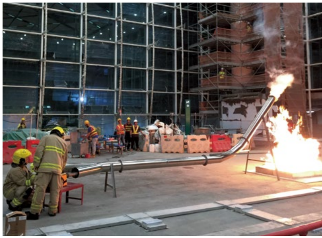
d. 消防处人员于机场一号客运大楼扩建部分进行检验巡查，确保其消防装置及设备的安装符合规格及运作正常。 The FSD personnel conduct acceptance inspection in the expanded Terminal 1 of Hong Kong International Airport to ensure proper installation and functioning of its FSIs and equipment.
